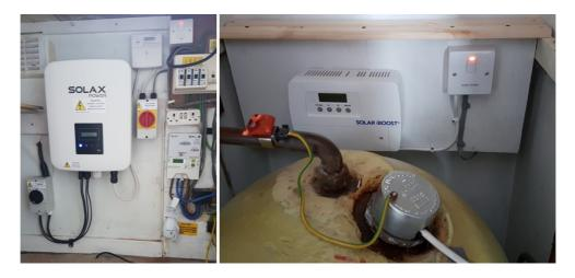
The best bit is the iBoost+ Buddy, its display tells you when the water is being heated and when the panels are not generating electricity.
